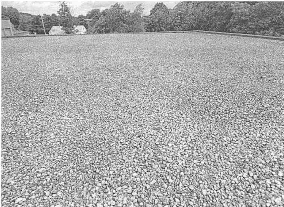
Overview of the roof system – Ballasted EPDM.
