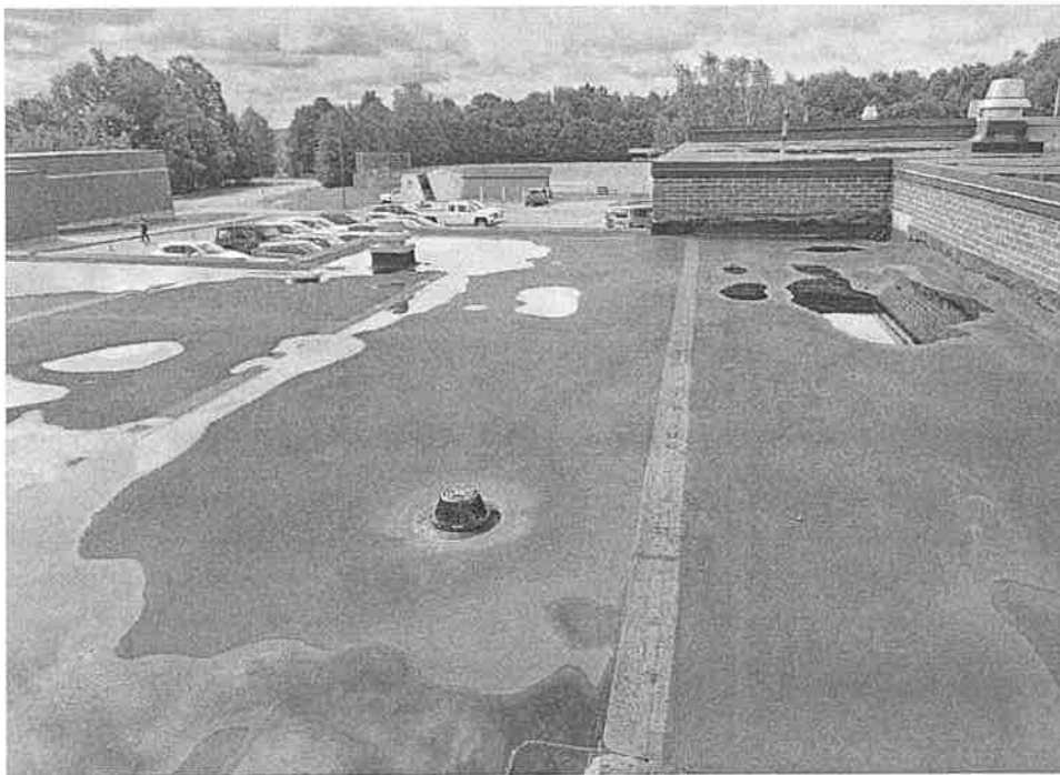
Overview of the roof system – Adhered EPDM.
