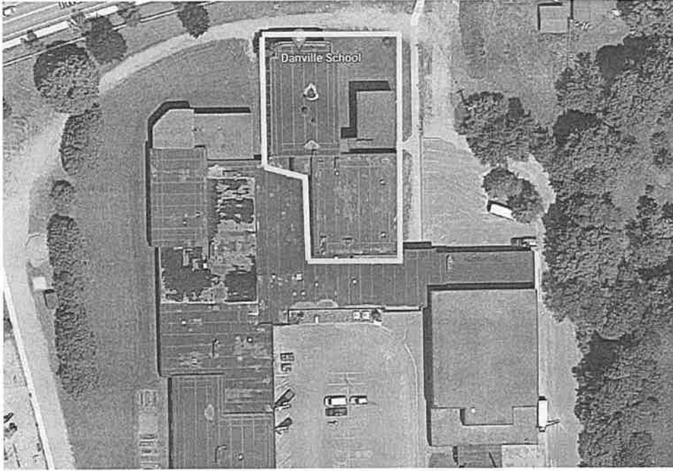
Roof area inspected.
