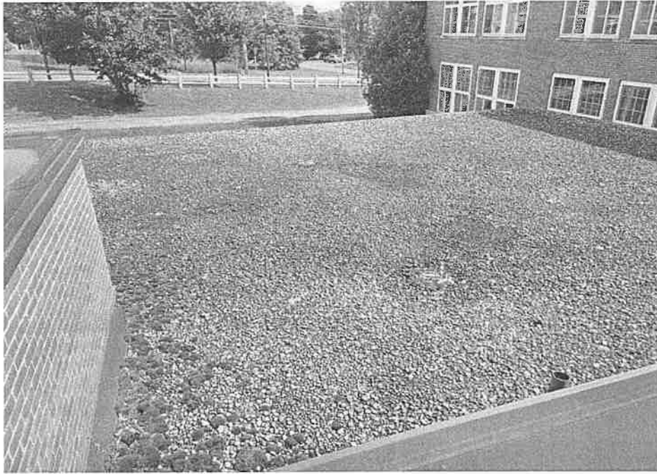
Overview of the roof system – Ballasted EPDM.
