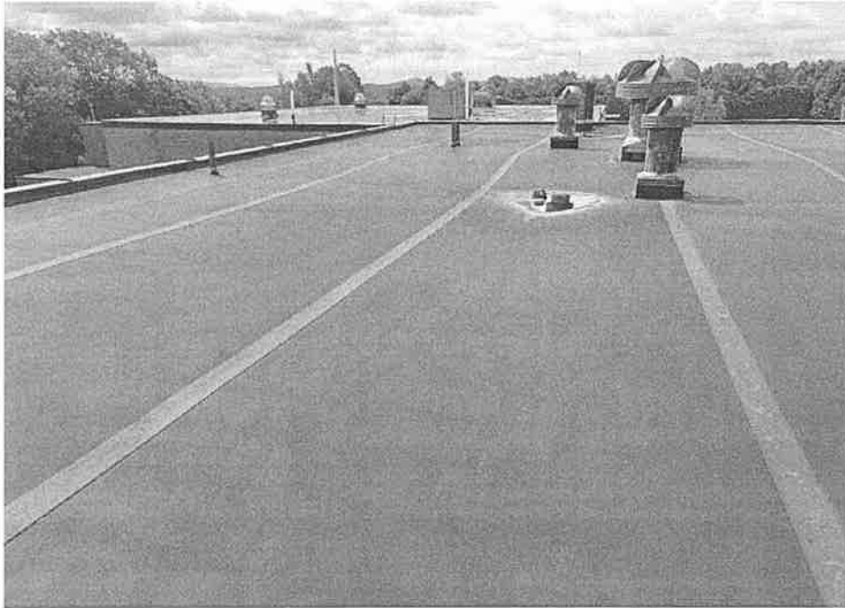
Overview of the roof system – Adhered EPDM.
