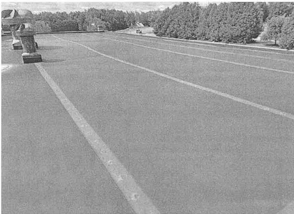
Overview of the roof system – Adhered EPDM.
