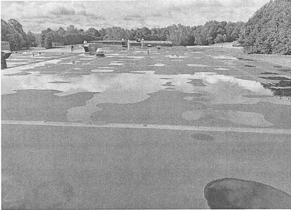
Overview of the roof system – Adhered EPDM.
