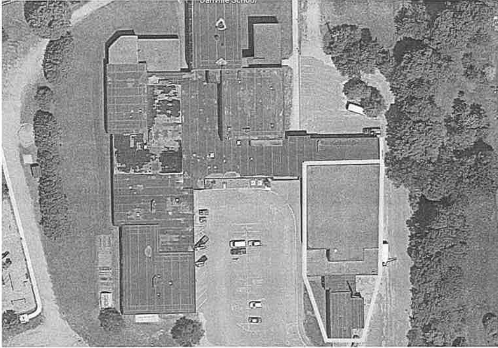
Roof area inspected.
