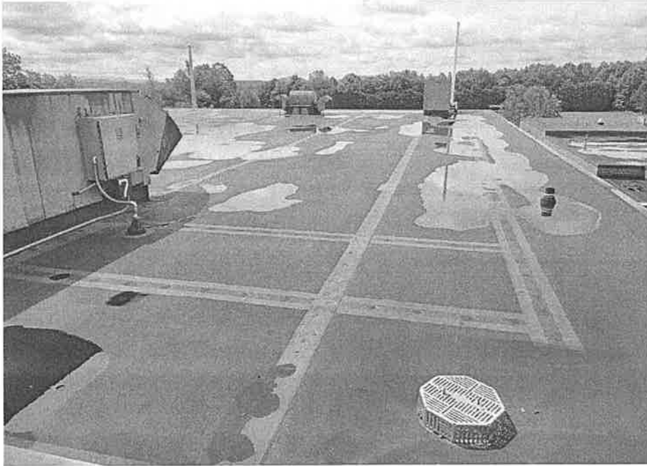
Overview of the roof system – Adhered EPDM.
