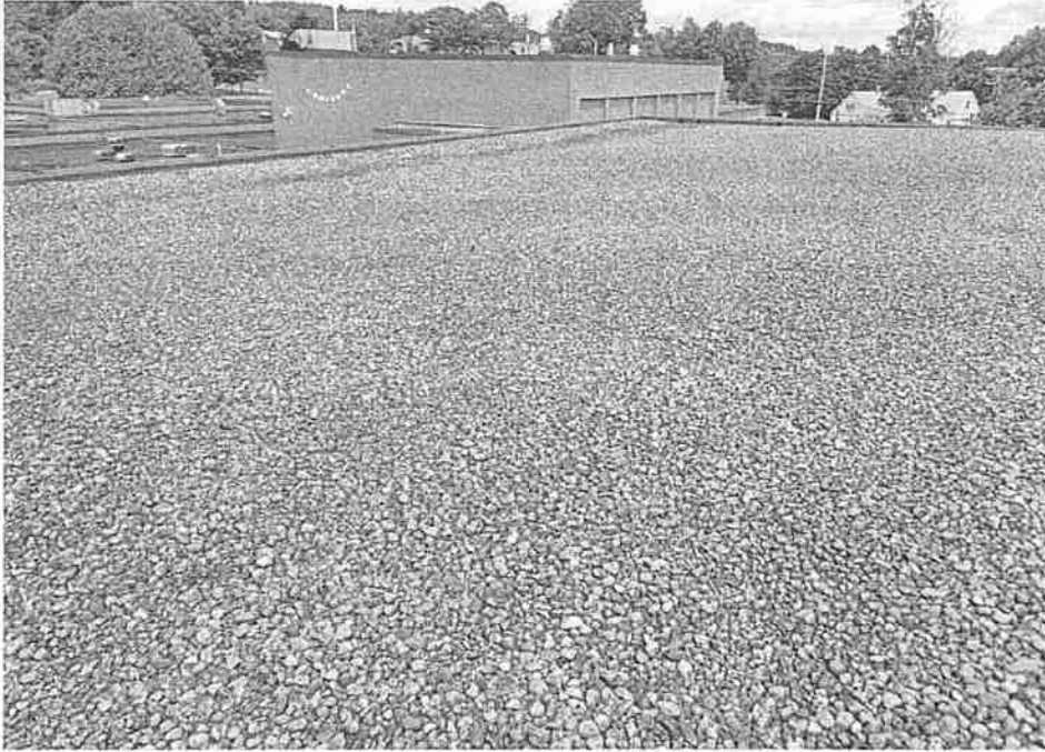
Overview of the roof system – Ballasted EPDM.
