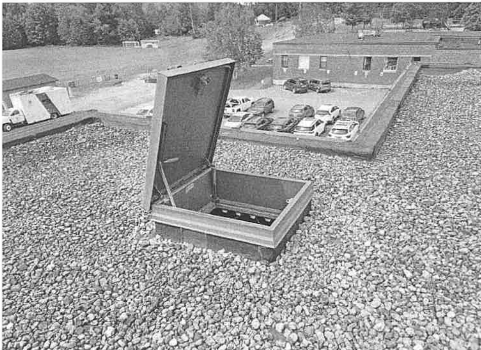
Roof access via internal hatch.
